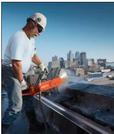
Husqvarna K750 Power Cutter's high-efficiency dual-charge 5hp engine delivers lower emissions and good fuel economy. © Photo courtesy of Husqvarna AB. Used with permission.
